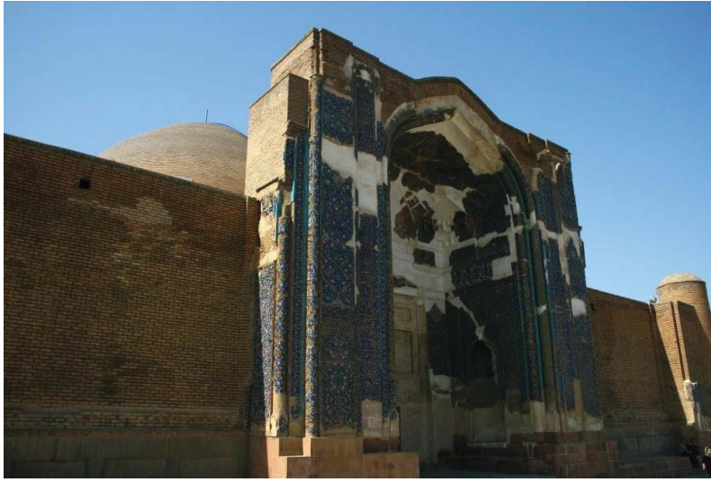
Picture 3 Gate of the Blue Mosque/ Masjid-i Kebud, Tabriz, 2015, (Photo: Akram Kazemipour Khabbazi).
